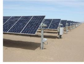
PV panels would either be crystalline silicon or thin film and would be well suited for the desert environment due to their durability and reliability. PV panels may be single-sided or bi-facial.
