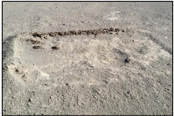
Figure 4 – One of the two contaminant barriers that has had the wood and plastic picked up but still has a small amount of contaminated soil to be disposed of.
