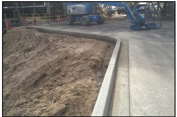
Figure 2 – Bull Concrete's freshly poured curb and gutter on the north side of the Power Block.
